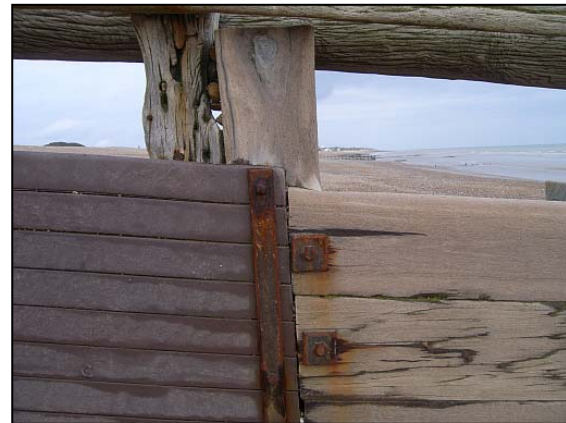
Comparative abrasion of plastic and wood at each end of the panel.
