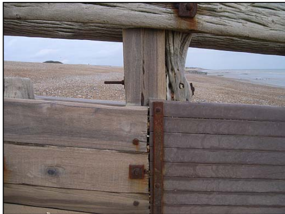
Comparative abrasion of plastic and wood at each end of the panel.
